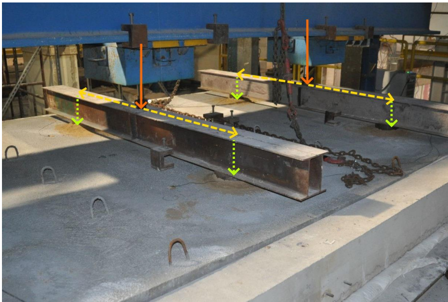
Fig. 2. Load distribution system (photo by: P. Turkowski, ITB)
