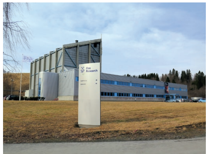
SP Fire Research AS in Trondheim.
