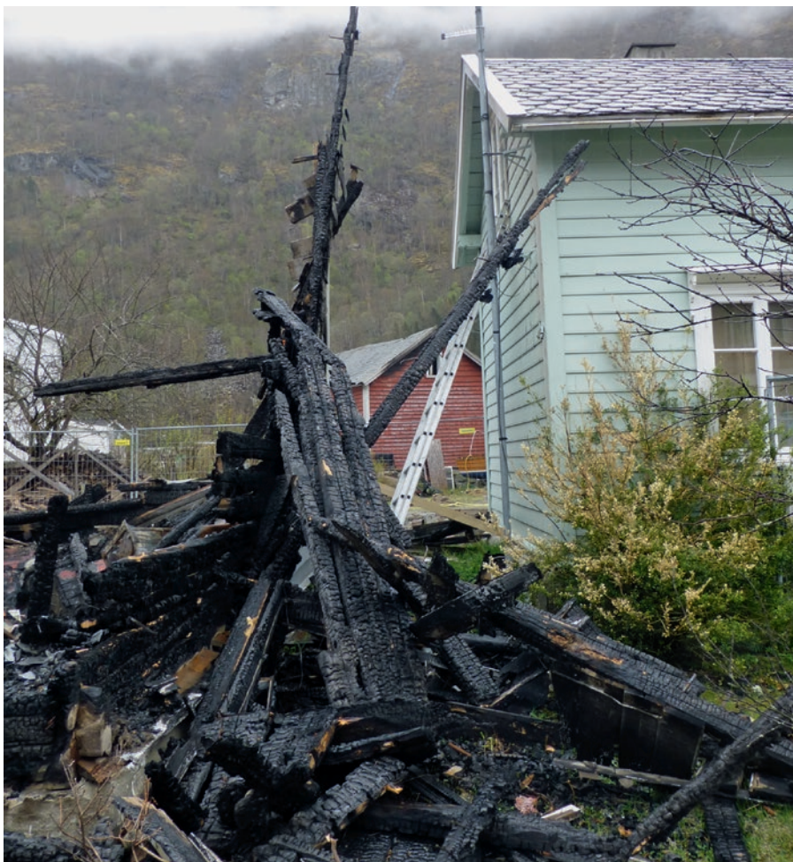
The house to the left was a protected wooden building from the 1840's, and was completely destroyed in the fire. The firefighters managed to save the protected house to the right from the flames. Photo: SP Fire Research AS.
